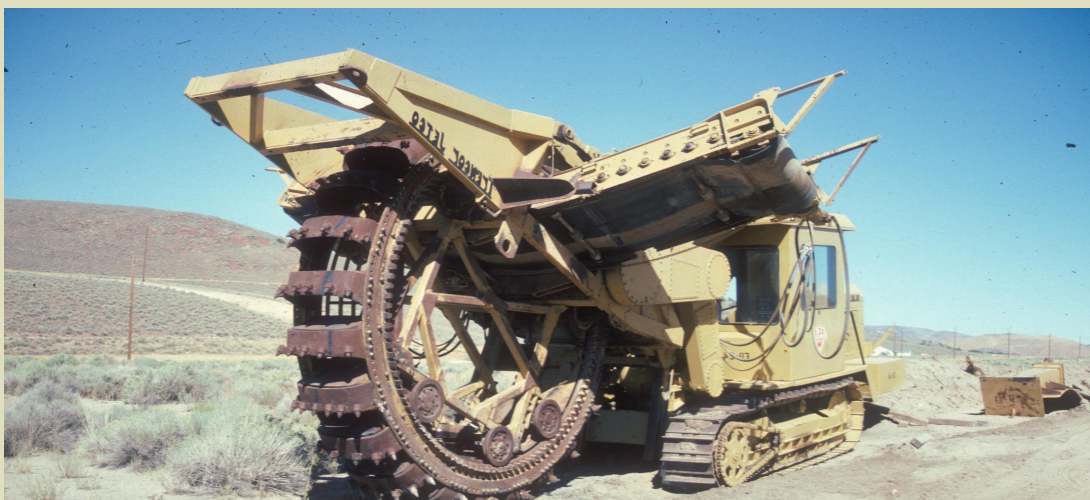
Figure 1. Heavy equipment used in pipeline construction is very visible as well as the disturbance.
